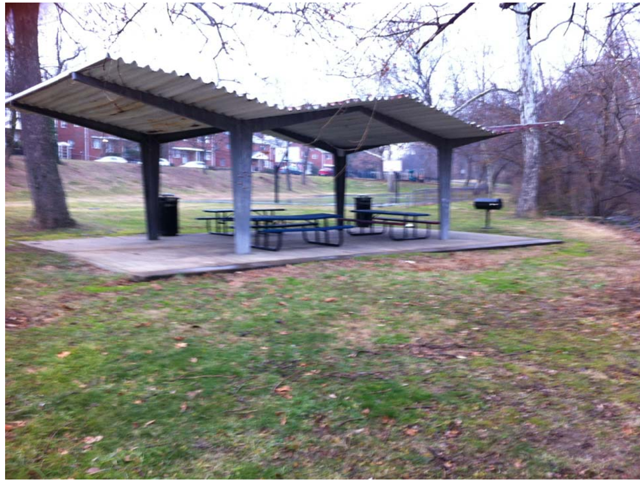
EX. PICNIC SHELTER , NORTHWEST, FACING VIEW
