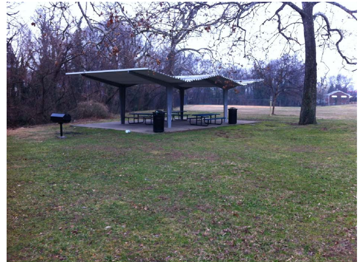
EX. PICNIC SHELTER , SOUTHEAST FACING VIEW
