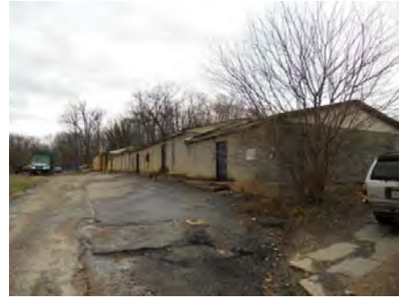
View of eastern end of warehouse located on northern portion of OWA (areas where removal of impacted soil are proposed are adjacent to warehouse).
