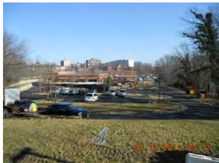
View from top FMM looking east towards JBM-HH maintenance facility.
