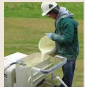
FIGURE 1: FILLING A PUMP WITH ORC ADVANCED SLURRY
