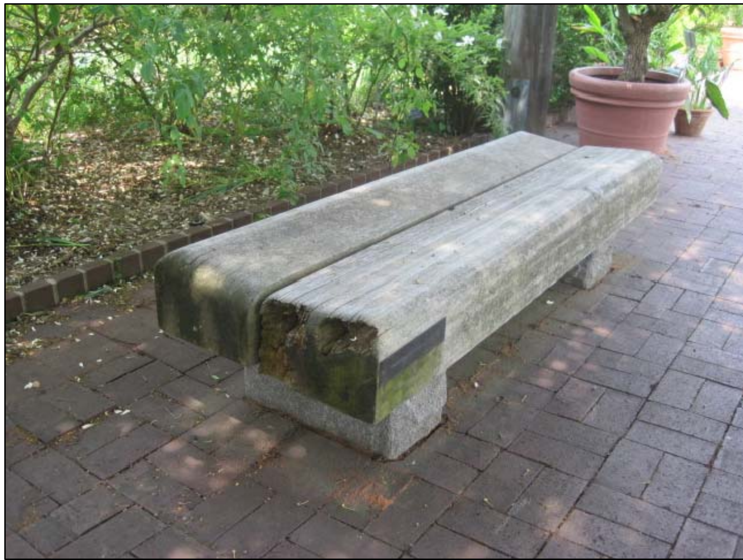
① EXISTING BENCH – REMOVE AND REPLACE WOOD COMPONENTS, BASE AND FOOTERS TO REMAIN NTS
