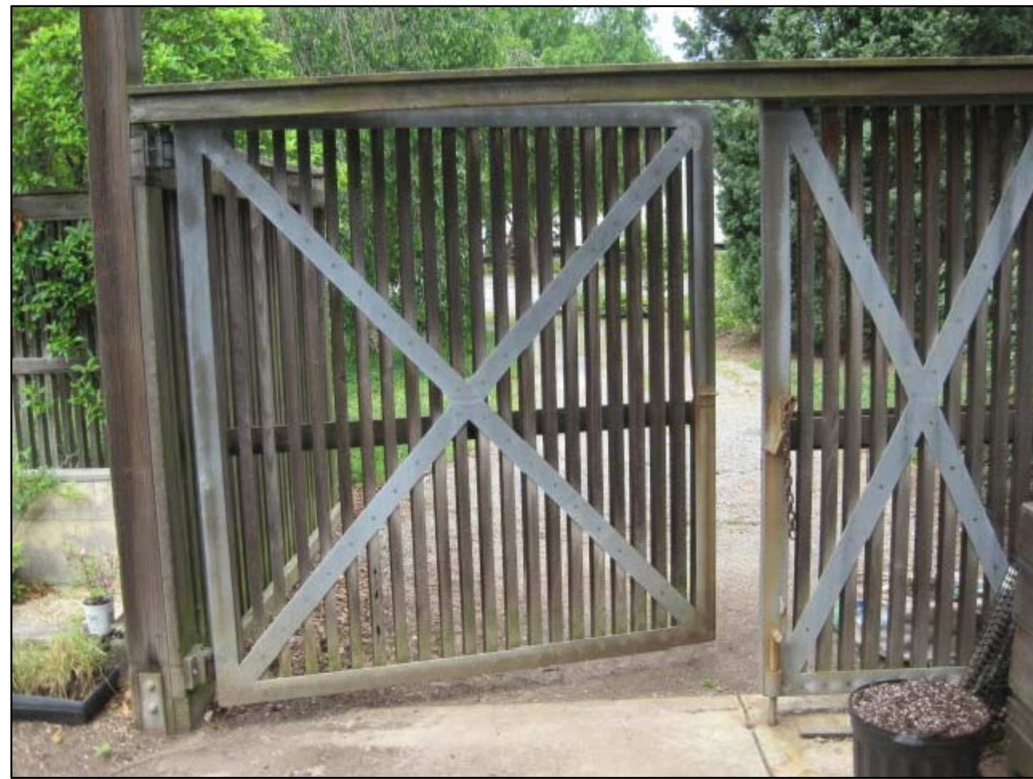
⑧ YARD GATES REMOVE AND REUSE METAL GATE FRAMES NTS
