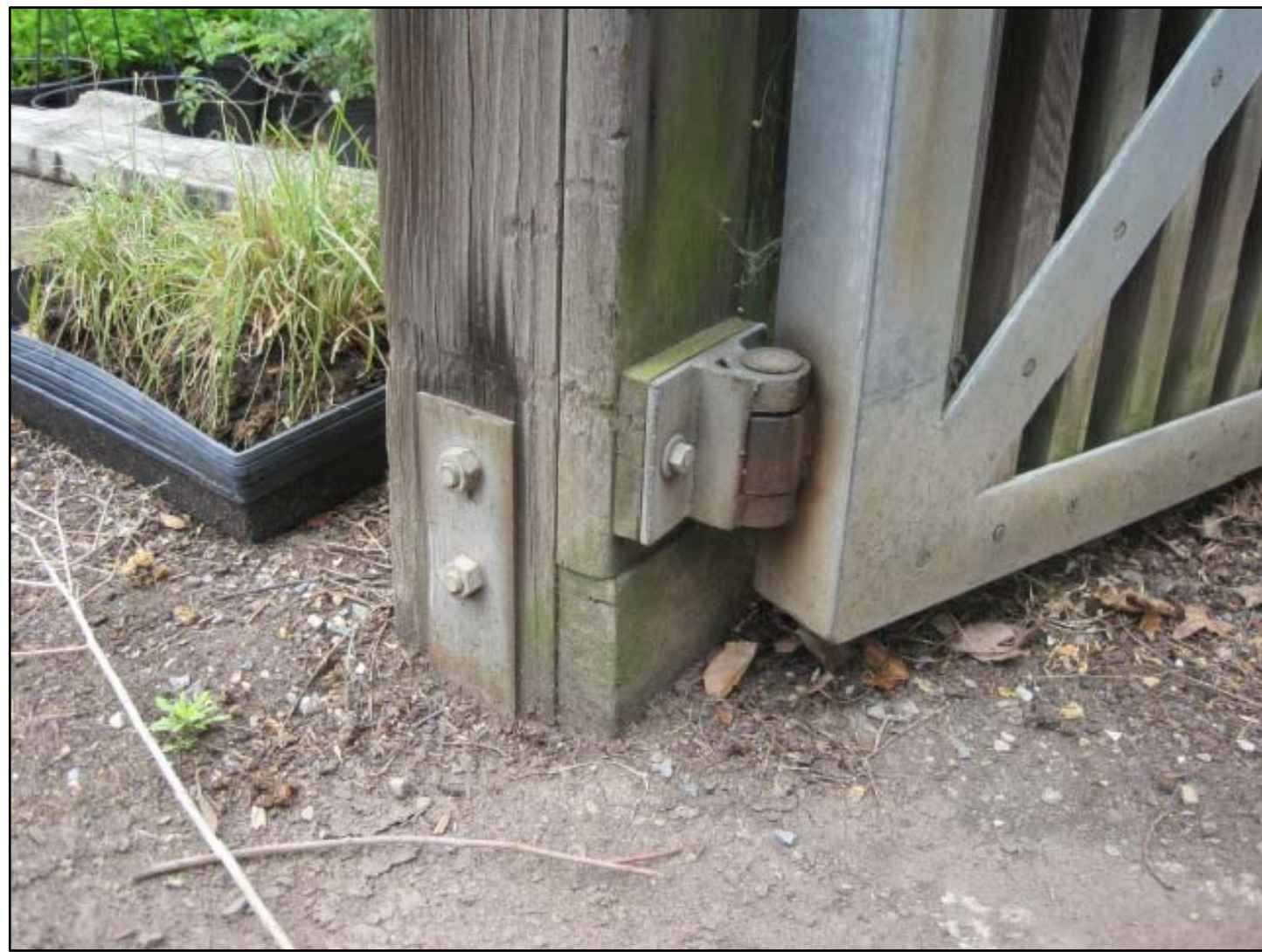
⑤ EXISTING YARD TRELLIS POST BRACKETS AND FOOTINGS TO REMAIN NTS
